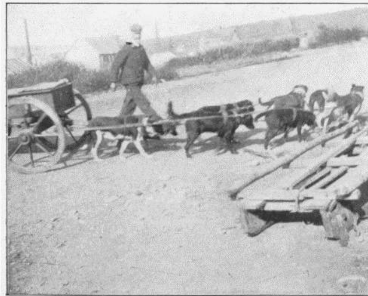
ATLIN CITY WATER WORKS.
