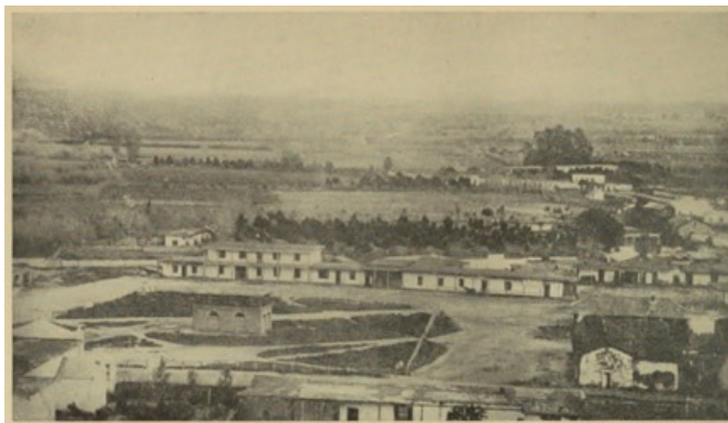
View of Plaza, Showing the Reservoir
