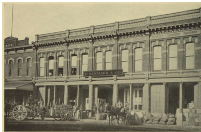
H. Newmark & Co.'s Building, Amestoy Block, about 1884
