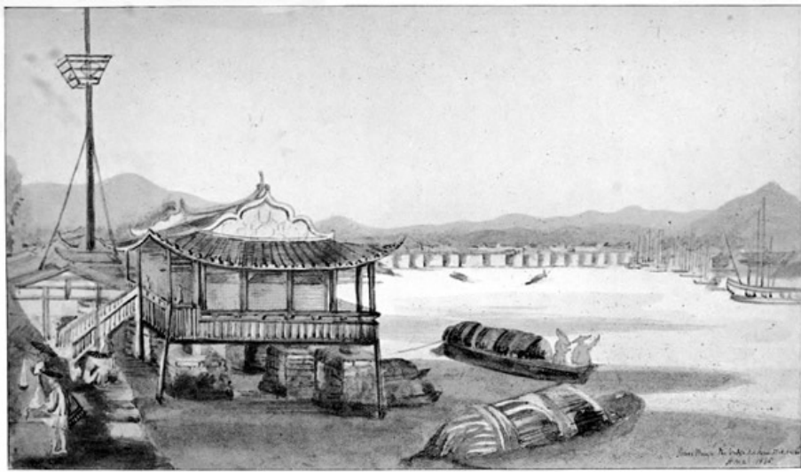
BRIDGE OVER RIVER MIN.
