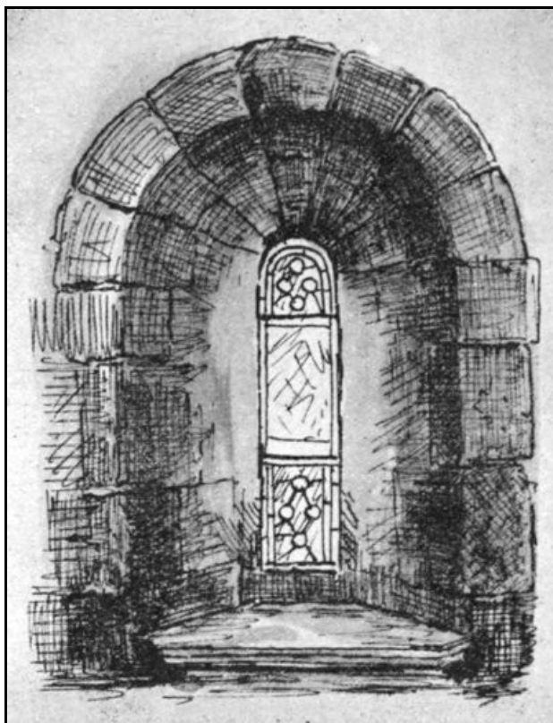
NORMAN WINDOW, WOODCHURCH, SHOWING WIDE SPLAY INSIDE
