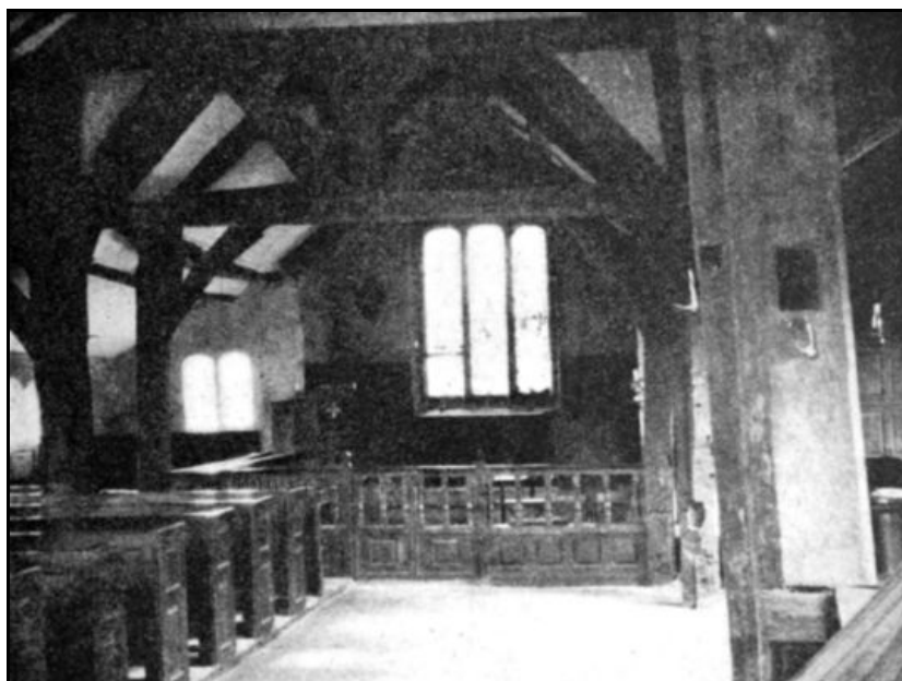
INTERIOR OF WARBURTON TIMBER CHURCH. FOURTEENTH CENTURY
