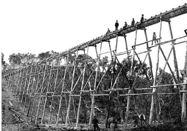
FIG. 9. FLUME, GREAT SOUTHERN GOLD-FIELD, SHOALHAVEN, N.S.W.
