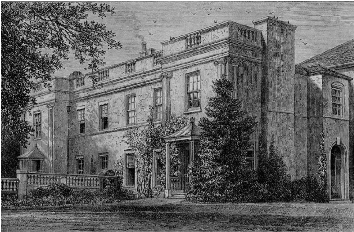
House in Folshill Road, Coventry."
