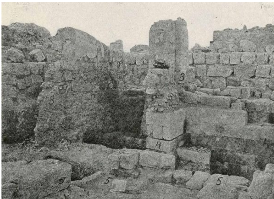
FIG. 42. WALLS OF BUILDINGS AT SAMARIA ( after Reisner ).
