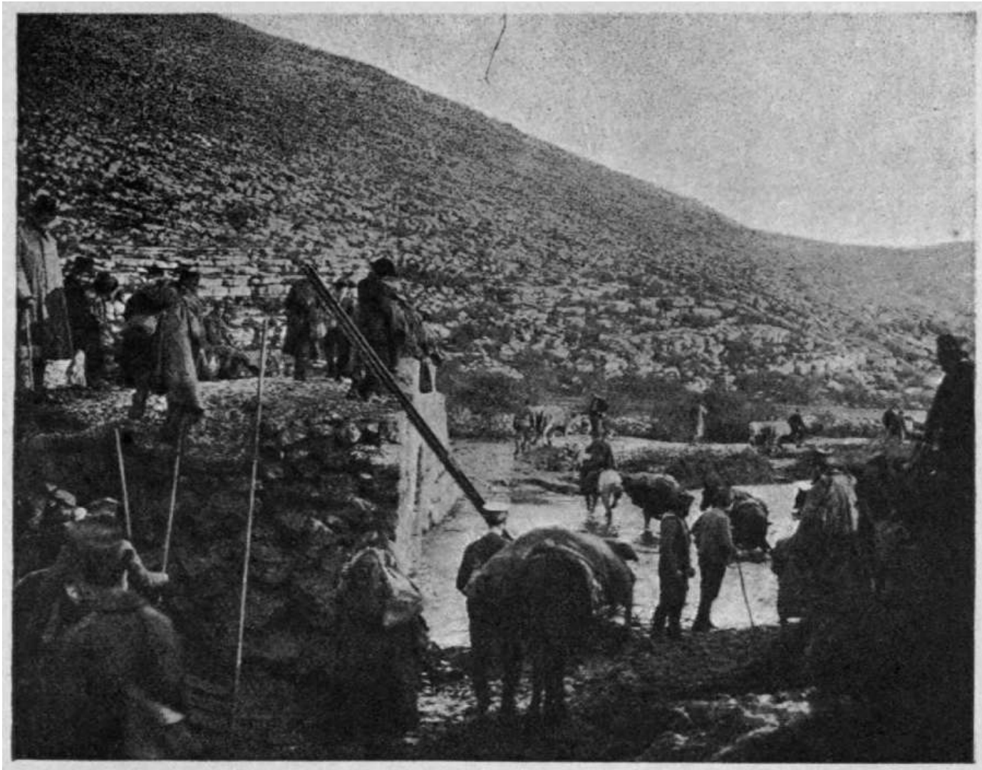
BROKEN BRIDGE AT FRONTIER BETWEEN MONTENEGRO AND ALBANIA Our route lay across the basaltic rocks
