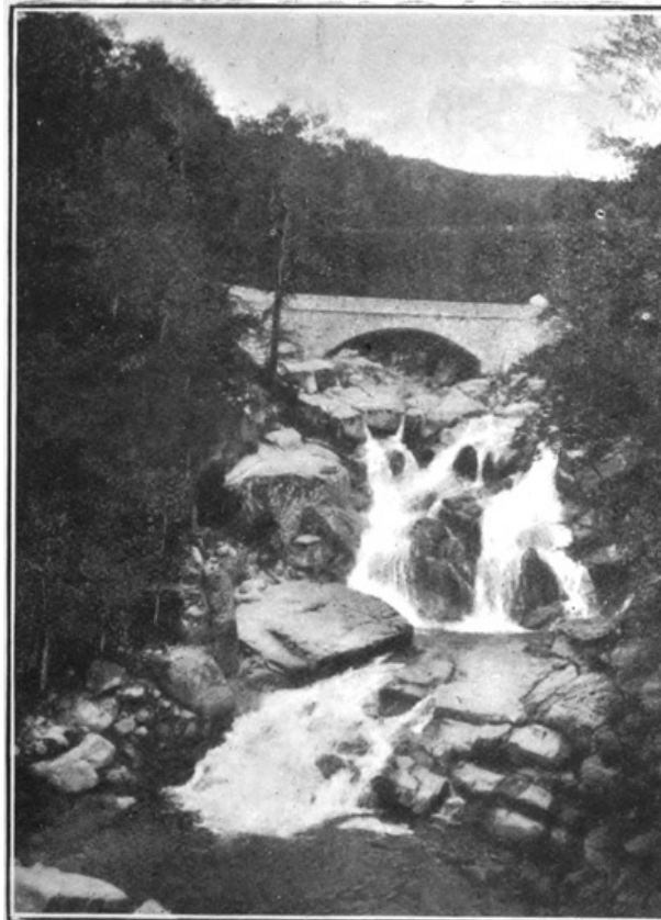
Waterfall on the Lozère, on Stevenson's route between Finiels and Pont de Montvert
