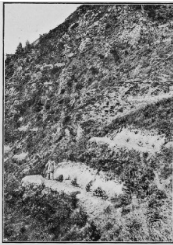
TERRACES CUT ON THE HILL SIDES AND PLANTED WITH TREES TO PREVENT THE FALL OF AVALANCHES. TO FACE P. 65.
