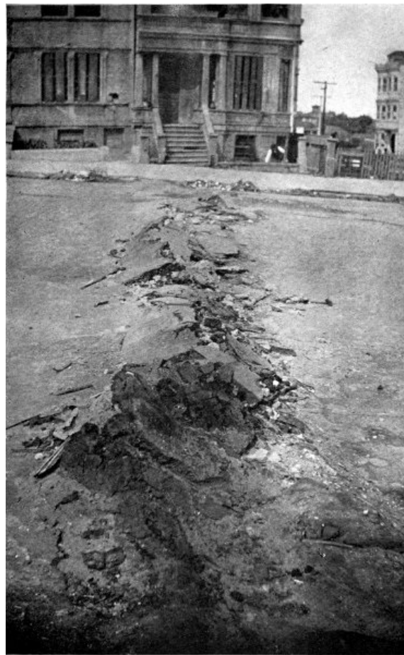
A SAN FRANCISCO PAVEMENT TORN BY THE EARTHQUAKE From a Stereograph, Copyright, 1906, by Underwood & Underwood
