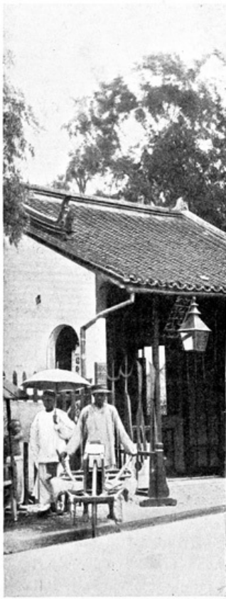
GUARD-HOUSE NEAR THE ARSENAL.
