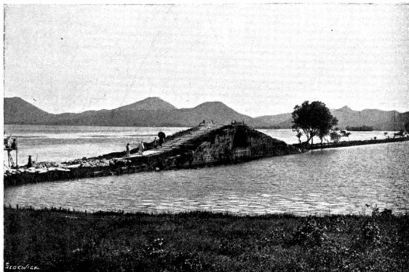
BRIDGE AND CAUSEWAY ON WEST LAKE.
