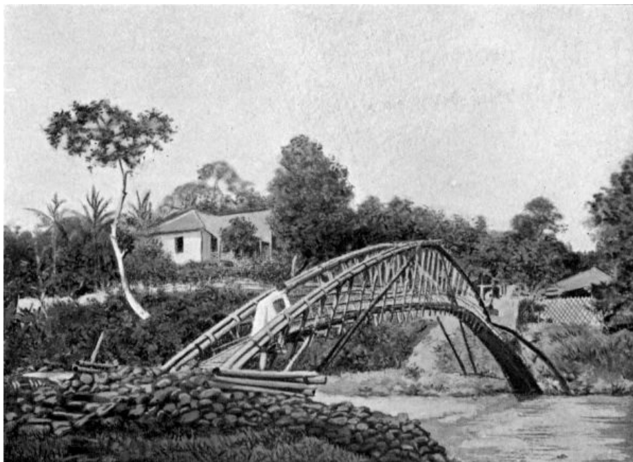
Bamboo bridge near Batu Tulis.
