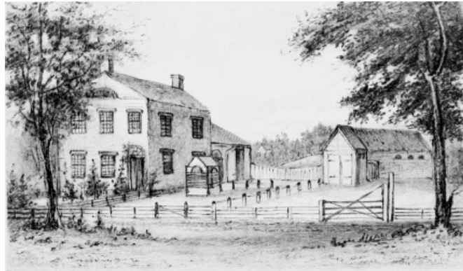
THE PARSONAGE, STOCKBRIDGE, MASS. (As rebuilt after the fire)
