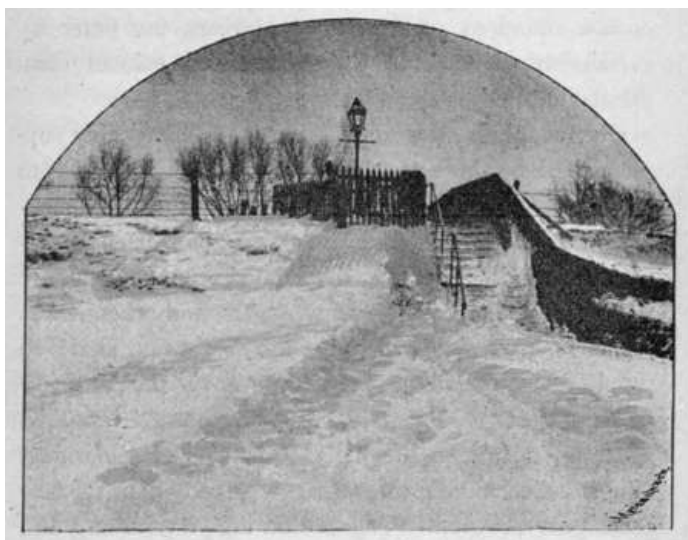
WATER STEPS, MILEHOUSE ROAD, DEVONPORT.
