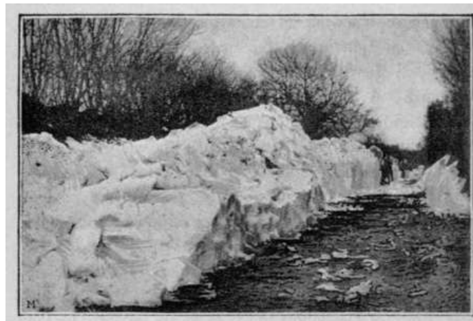
CUTTING A ROAD AT BRENT.
