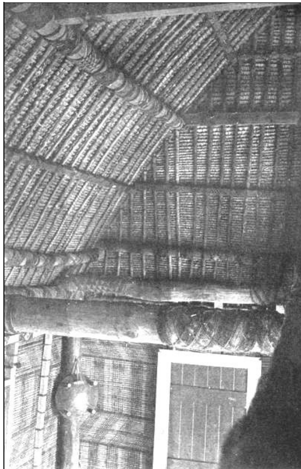
INTERIOR OF FIJIAN HOUSE, SHOWING HOW IT IS BOUND
