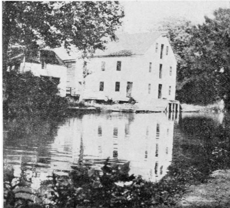
Above—Upper Level at Four Locks Below—Old-Time Mill
