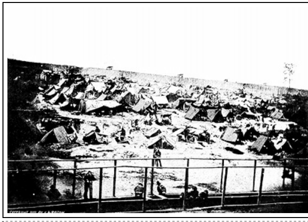
ANDERSONVILLE PRISON WITH ITS STOCKADE AND GUARD TOWERS
