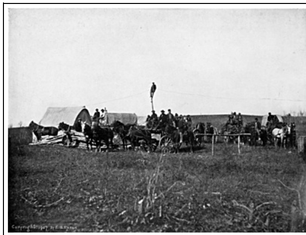
PHOTOGRAPH TAKEN AS MILITARY TELEGRAPH WAS BEING STRUNG
