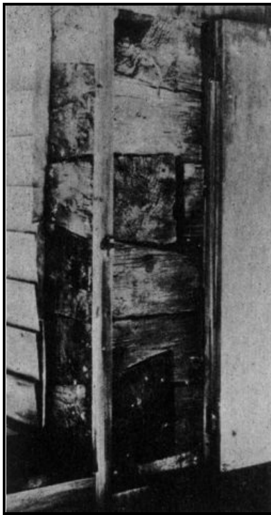
CORNER OF THE MCINTYRE GARRISON HOUSE, NEAR YORK, ME.
