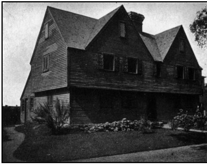
THE JOHN WARD HOUSE, SALEM. BUILT IN 1684 Showing overhanging second story, gable windows and casement sash
