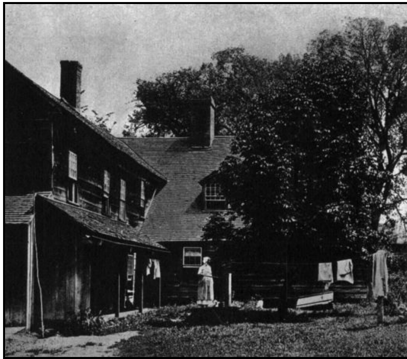
REAR OF THE SAXTON HOUSE, DEERFIELD, MASS. Showing unpainted weatherboarding
