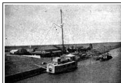
Signalstation am Suez-Kanal.
