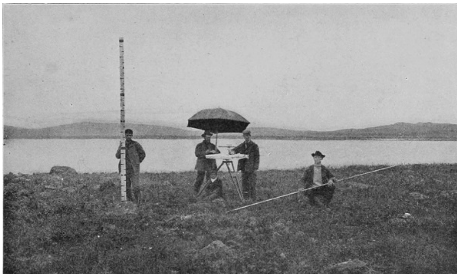
FIG. 11. TOPOGRAPHIC SURVEY PARTY AT WORK WITH PLANE TABLE ON THE PRIBILOF ISLANDS.
