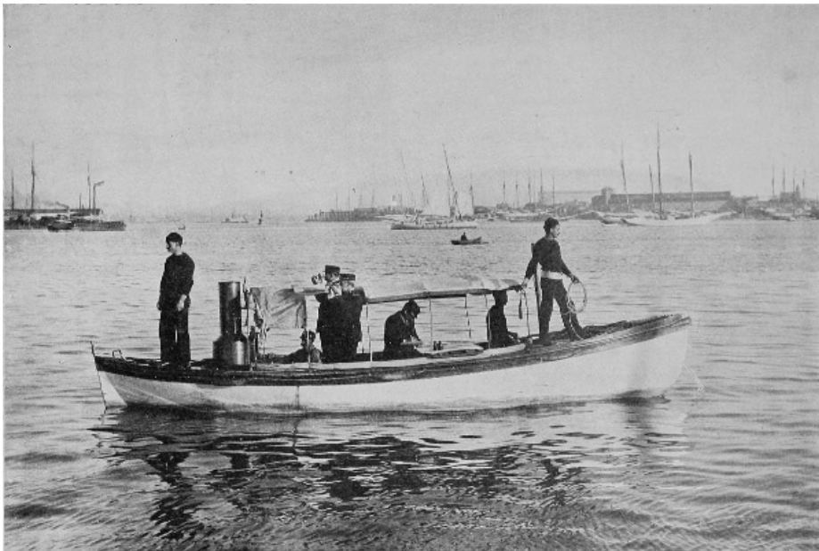
FIG. 13. HYDROGRAPHIC PARTY SOUNDING WITH LAUNCH IN BALTIMORE HARBOR.
