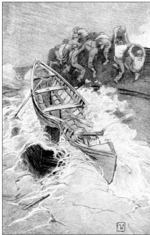
Saving the Cylinder of the Lighthouse at Smith Point, Chesapeake Bay, from being Swamped in a High Sea.
