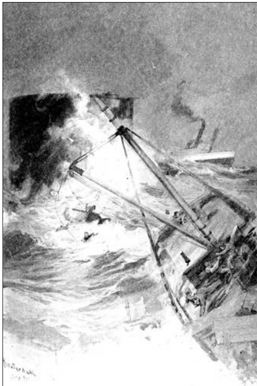
Work on the Smith Point Lighthouse Stopped by a Violent Storm.
