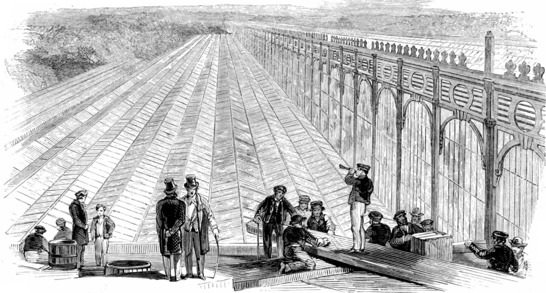
View of Glass Roof from the Lead Flat.
