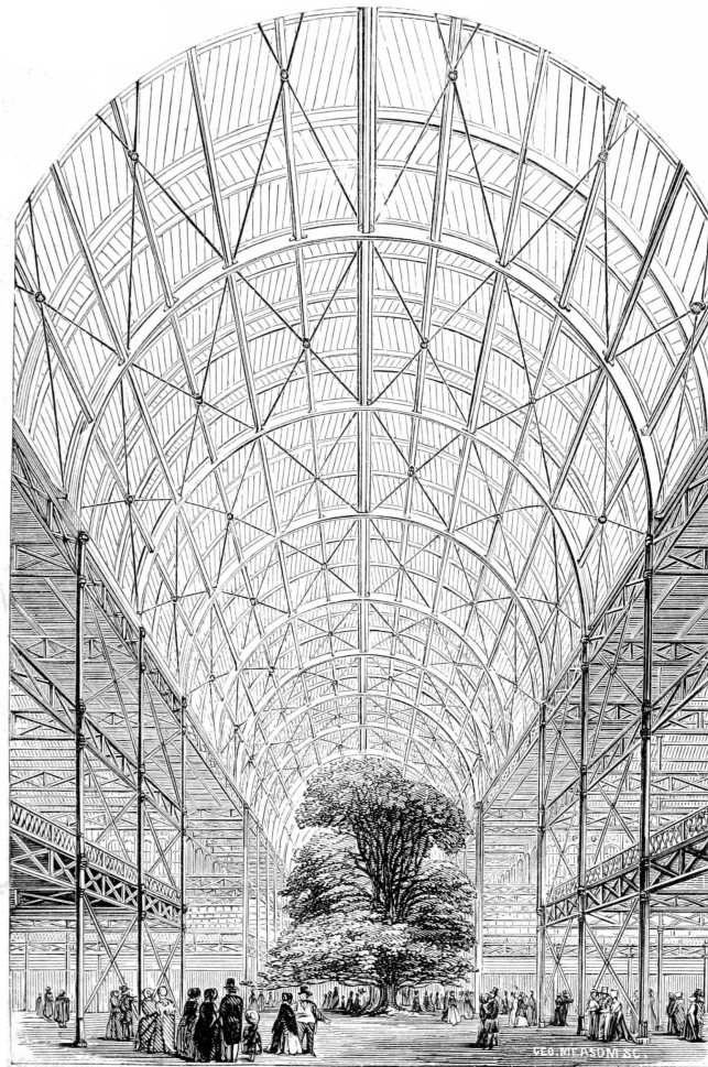
View of the Interior of the Transept.
