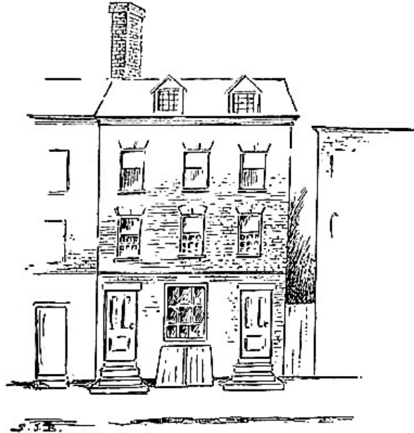
HOUSE AT 122 WILLIAM STREET
