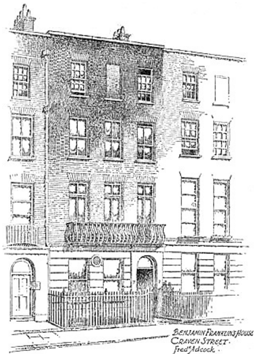
BENJAMIN FRANKLIN'S HOUSE. CRAVEN STREET.
