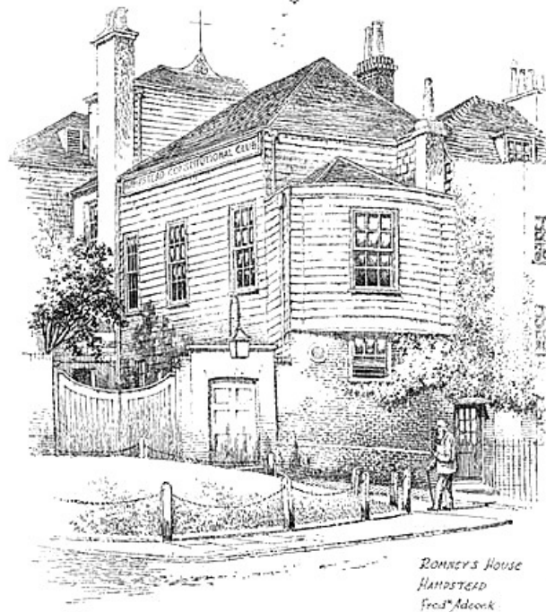
ROMNEY'S HOUSE. HAMPSTEAD.
