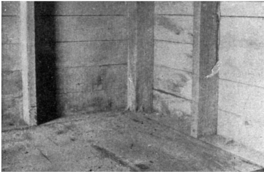
The flooring must be perfectly tight to prevent drafts coming through it
