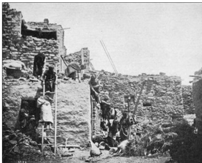
HOPi WOMEN BUILDING A HOUSE AT ORAIBI.
