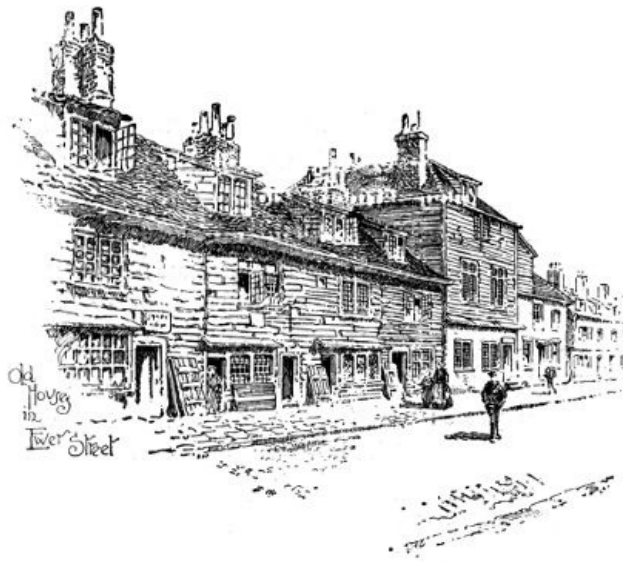
Old Houses in Ewer Street
