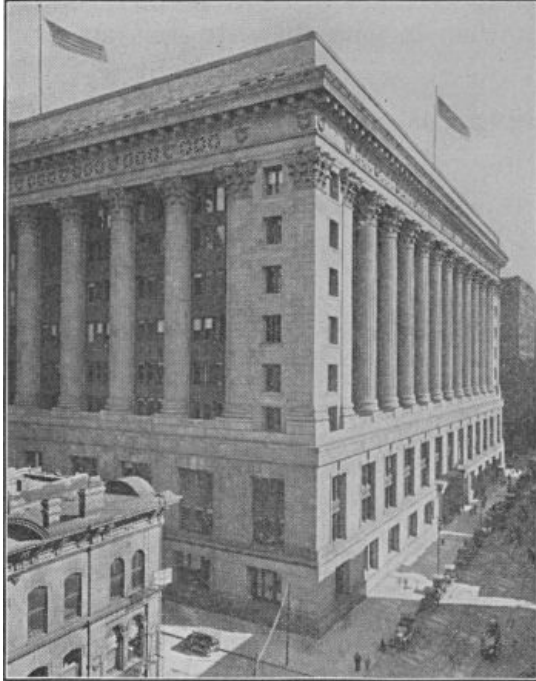
COURTHOUSE AND CITY HALL
