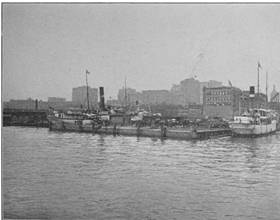
ONE OF THE NEW WHARVES
