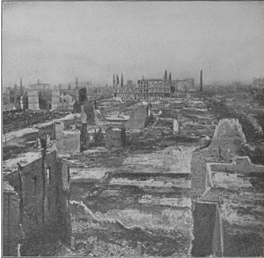
AFTER THE FIRE
