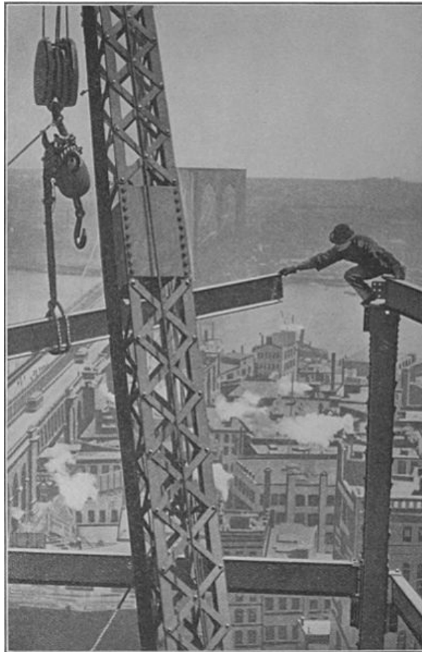
BUILDING A SKYSCRAPER
