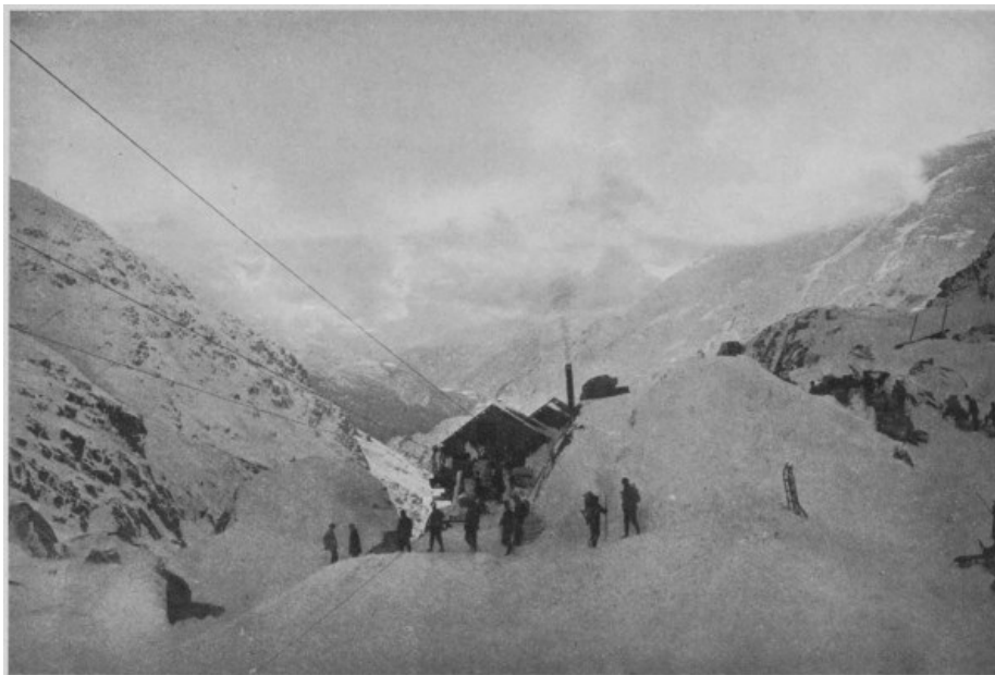
THE CHILKOOT TRAIL—POWER HOUSE OF THE AÉRIAL TRAMWAY.
