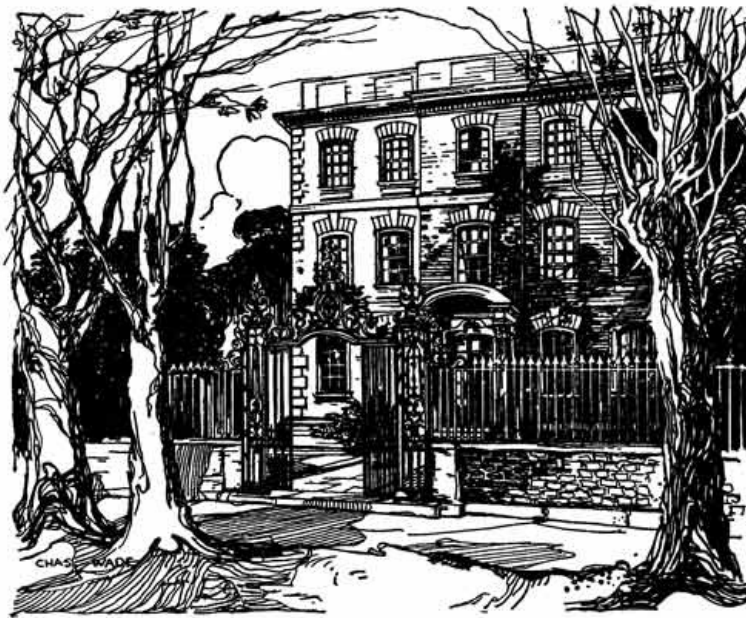
House at Rainham, Essex, built during the reign of Queen Anne
