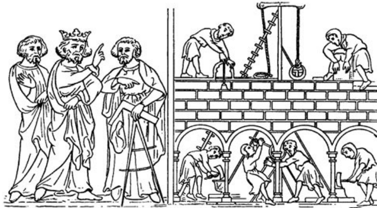
Foundation of a Minster
