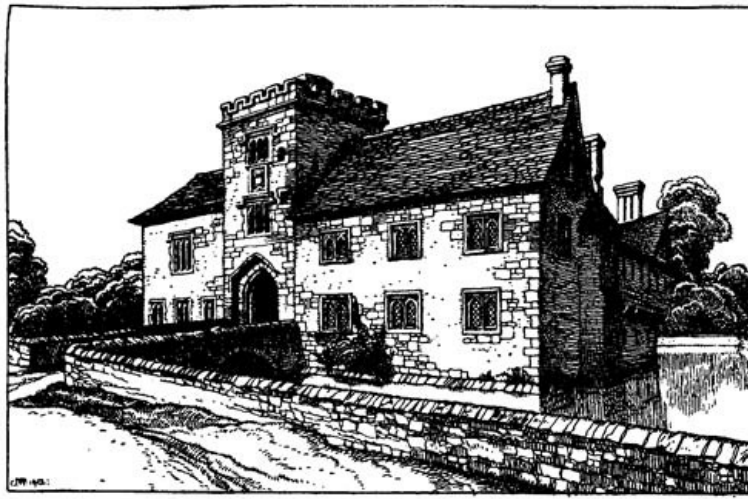
The Moat House, Ightham, Kent. An example of a fortified manor house of feudal times. A large portion appears to be work of the fourteenth century
