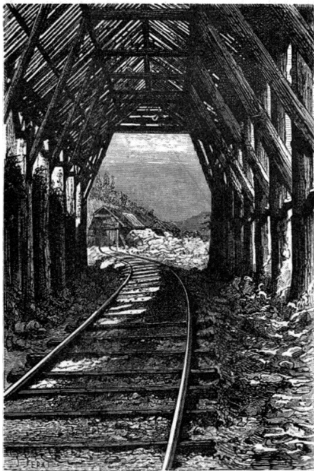
ON THE PACIFIC RAILWAY: THE INTERIOR OF A SNOW-SHED IN THE SIERRA NEVADA.
