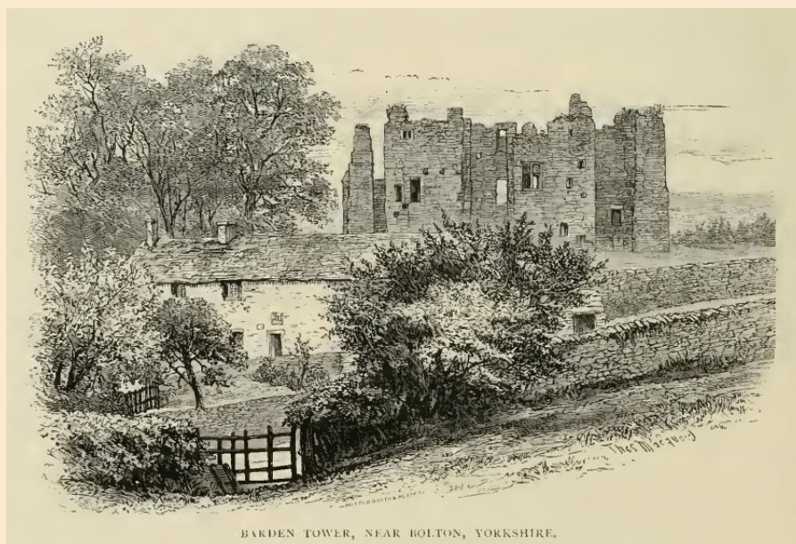
BAKDEN TOWER, NEAR BOLTON, YORKSHIRE.
