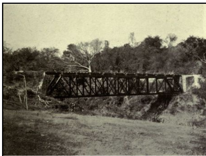
DECK BRIDGE ON SALVADOR RAILWAY.
