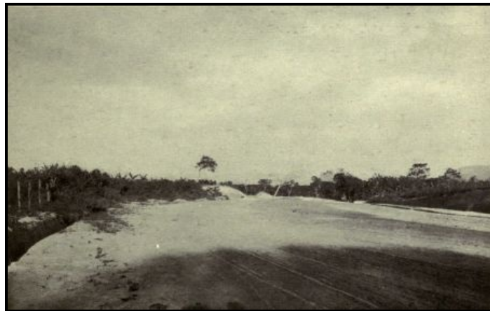
THE FAMOUS AVENIDA UNDER CONSTRUCTION.
