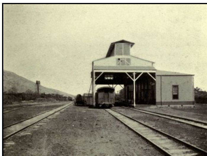
STATION BUILDING AT SANTA ANA ON THE SALVADOR RAILWAY.
