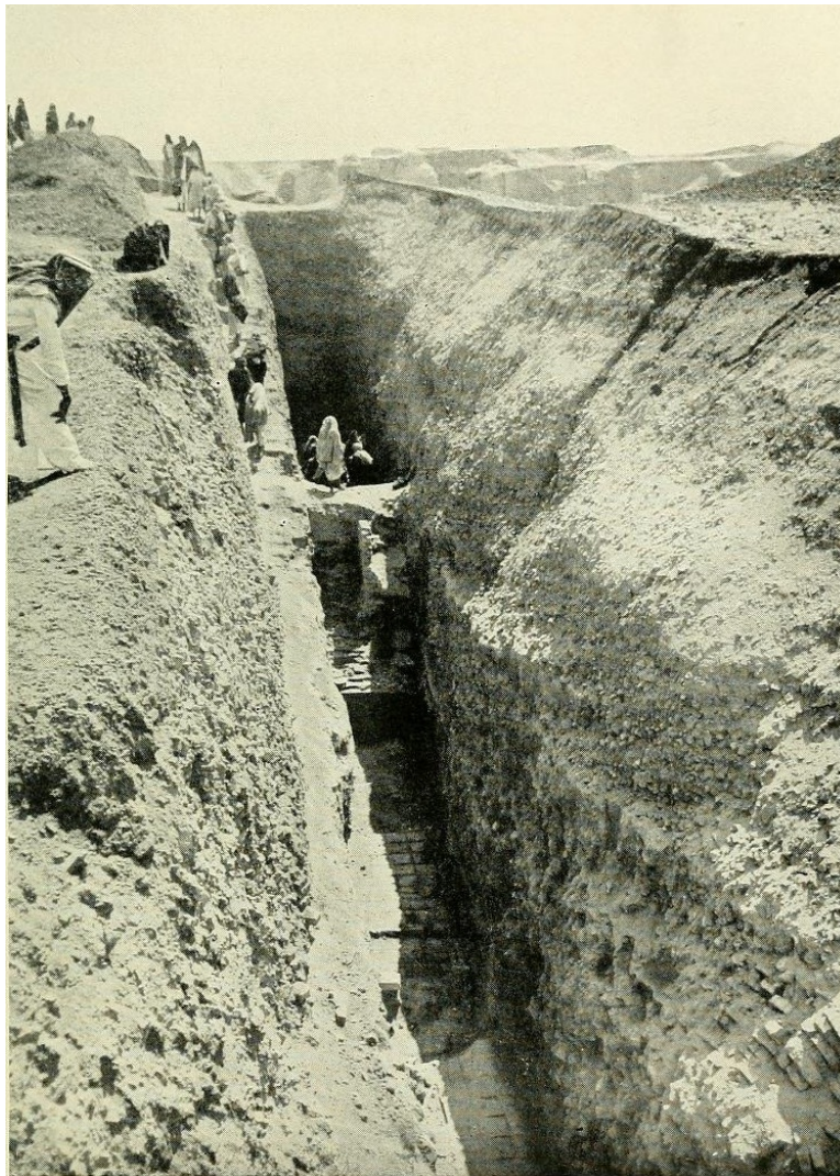
Work of the excavators in Babylon. One hundred workmen laboured in digging this cut, which is 40 feet deep. Copyright by Underwood and Underwood, London.
