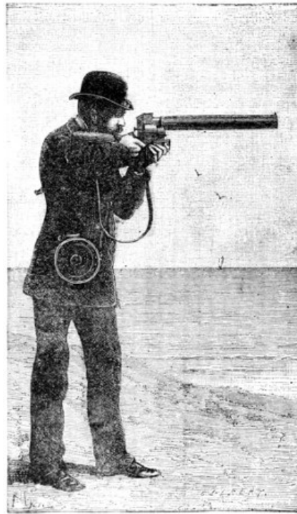
FIG. 17.—MODE OF USING THE PHOTOGRAPHIC GUN.
