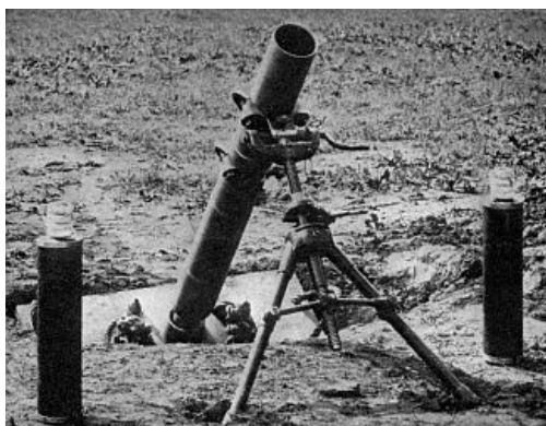
A 3-inch Stokes mortar and two of its shells
