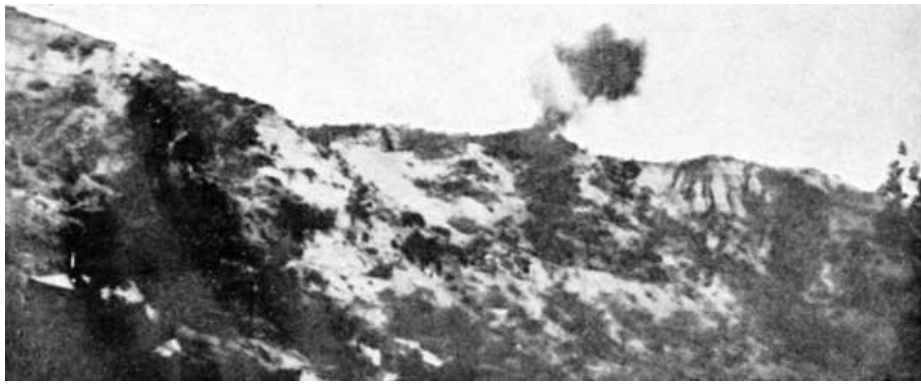
A SHELL BURST ON STEEL'S POST.
