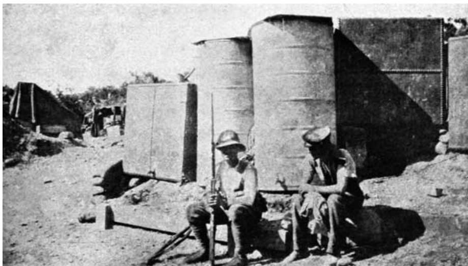
A MAORI ON SENTRY AT THE WATER TANKS IN MULE GULLY.
