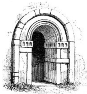
Saxon Doorway (Tower of Earls-Barton Church)
