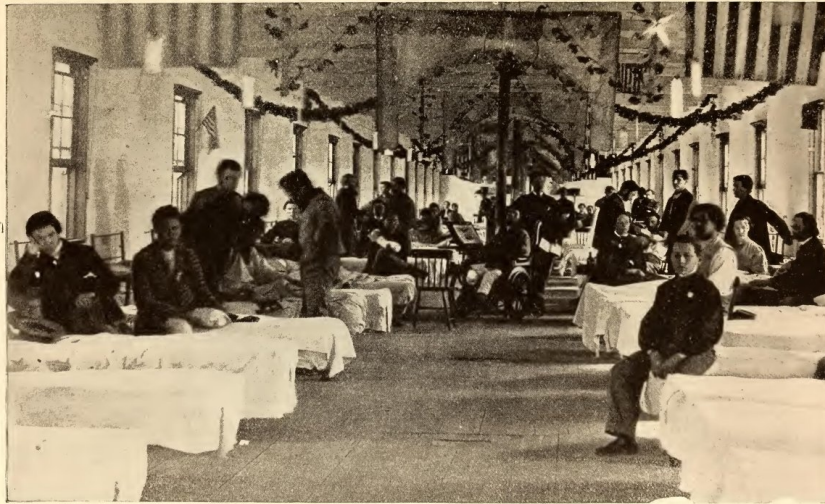
INTERIOR OF HOSPITAL—CONSTRUCTED BY THE SANITARY COMMISSION.
