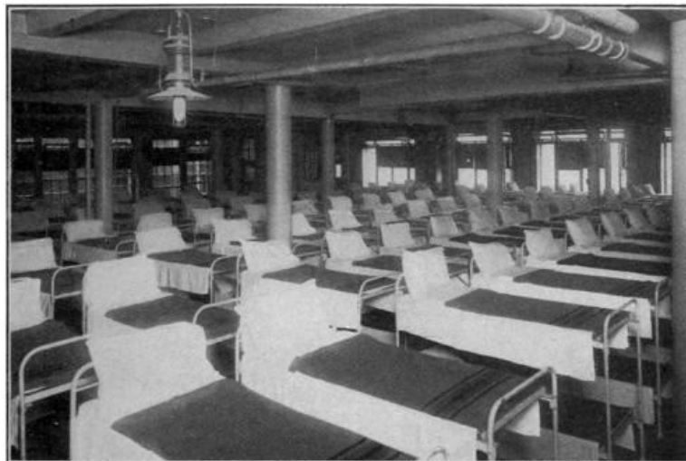
MUNICIPAL Lodging House, New York City Male Dormitory
