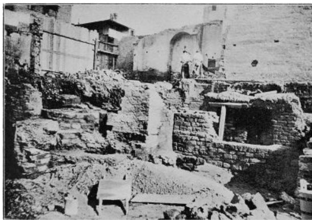
EXTERIOR VIEW OF CALIDARIUM AND FURNACE.
