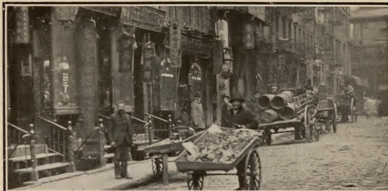
PELL STREET, THE NORTHERN BOUNDARY OF CHUCK CONNORS' "RESERVATION."
