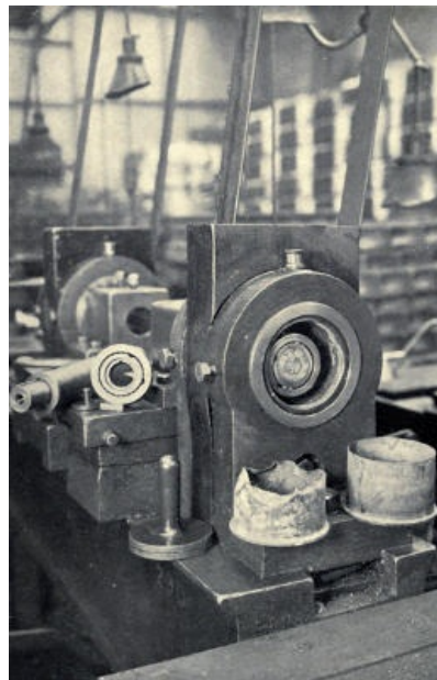
ROLLING OUT DENTS IN 4.5-INCH FIRED CARTRIDGE CASE.
