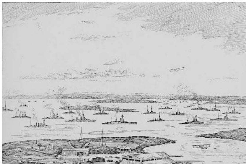
VIEW LOOKING SOUTH FROM HOUTON BAY.
