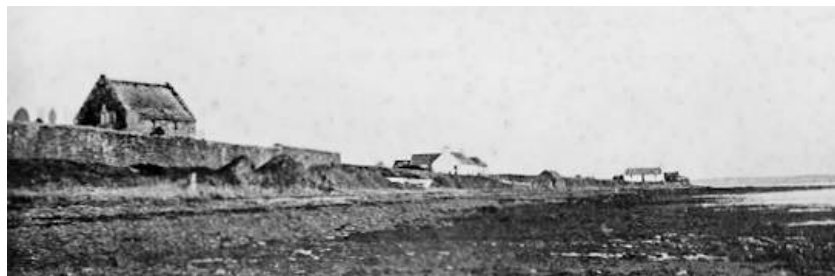
KIRK HOPE, SOUTH WALLS.
