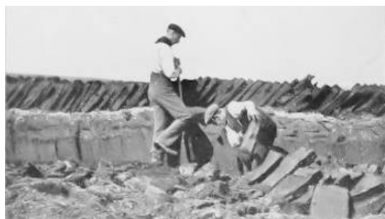
DIGGING THE PEATS—HOY.
