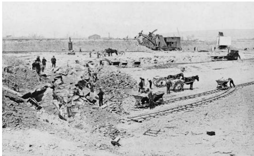
EXCAVATIONS AT LYNESS IN CONNECTION WITH THE BUILDING OF THE WHARF.
