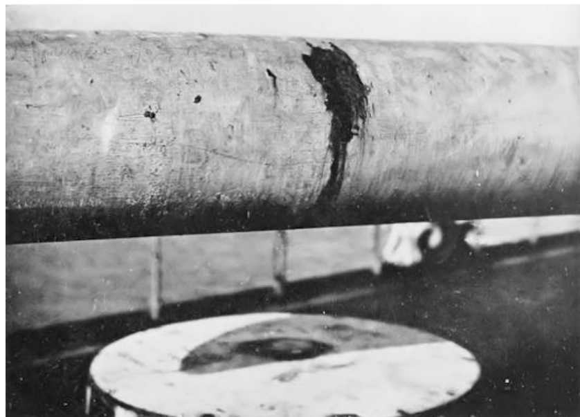
EXPANSION RING MARKING ON 6-INCH GUN "NURNBERG."
