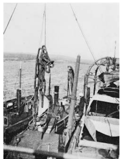
LIFTING CHAIN CABLES.
