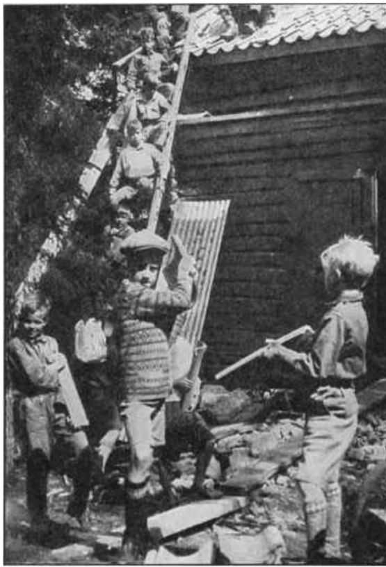
NILS HELPING TO REPAIR THE ROOF
