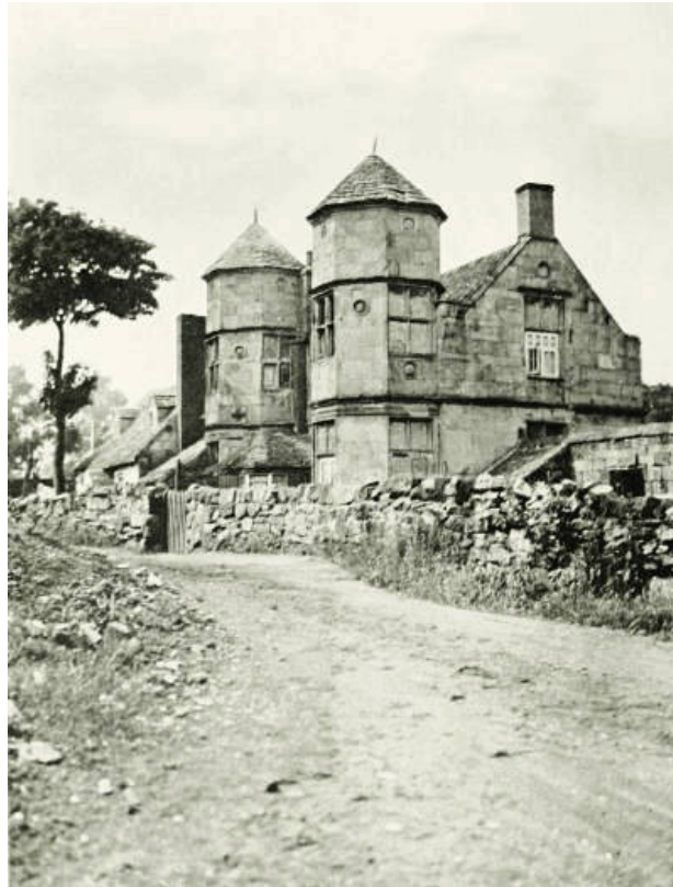
MADELEY COURT, GATEHOUSE.
