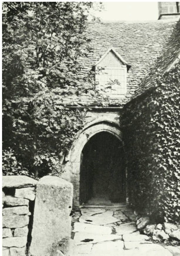
A FOURTEENTH-CENTURY DOORWAY.
