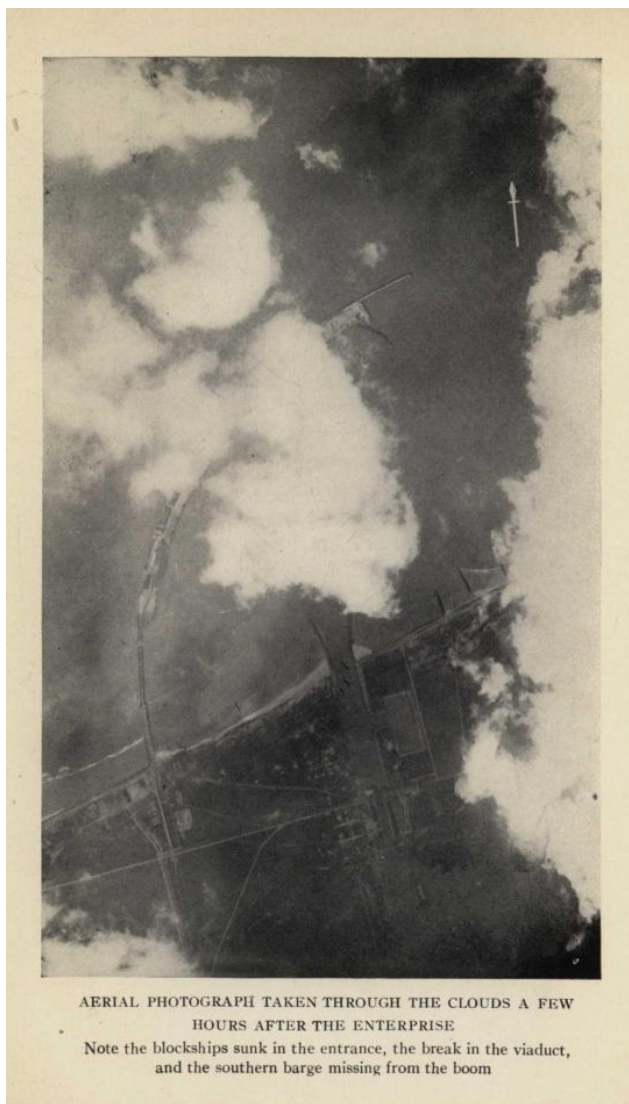
AERIAL PHOTOGRAPH TAKEN THROUGH THE CLOUDS A FEW HOURS AFTER THE ENTERPRISE. Note the blockships sunk in the entrance, the break in the viaduct, and the southern barge missing from the boom.
