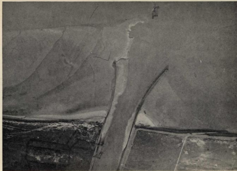
AERIAL PHOTOGRAPH OF THE CANAL ENTRANCE
