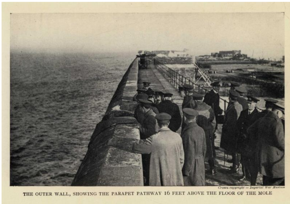
THE OUTER WALL, SHOWING THE PARAPET PATHWAY 16 FEET ABOVE THE FLOOR OF THE MOLE
