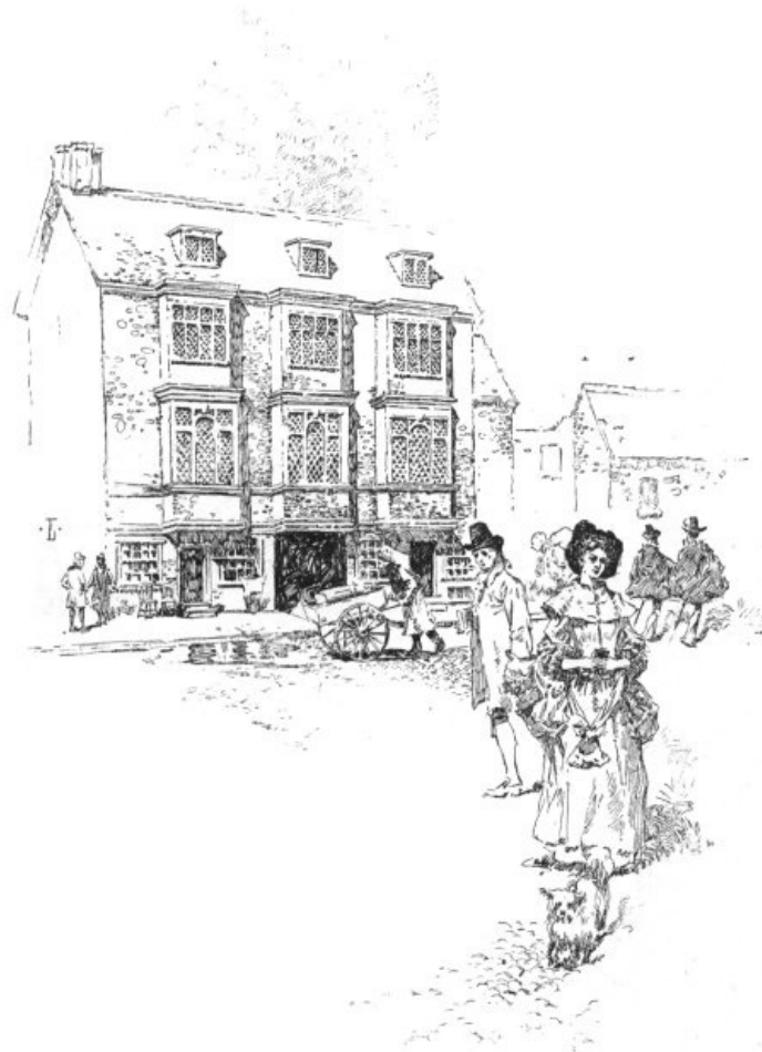
SOUTH VIEW OF FALCON TAVERN, ON THE BANK SIDE, SOUTHWARK, AS IT APPEARED IN 1805
