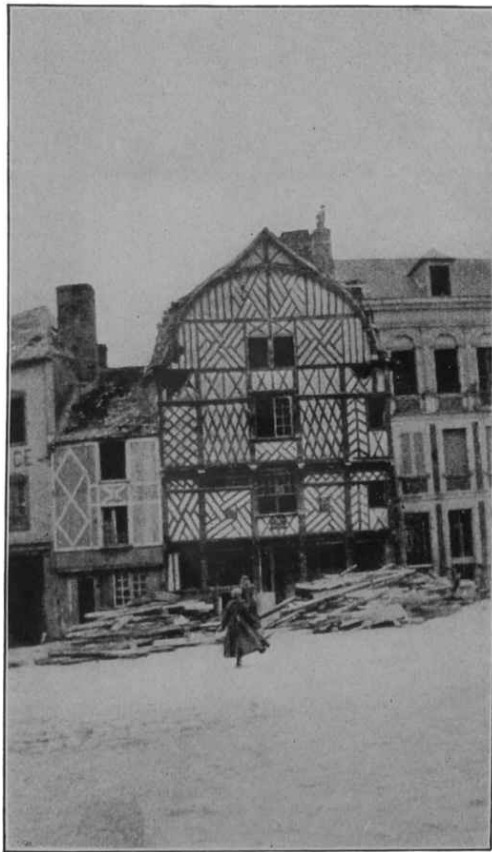
Very Old and Beautiful House at Roye Interior completely gone
